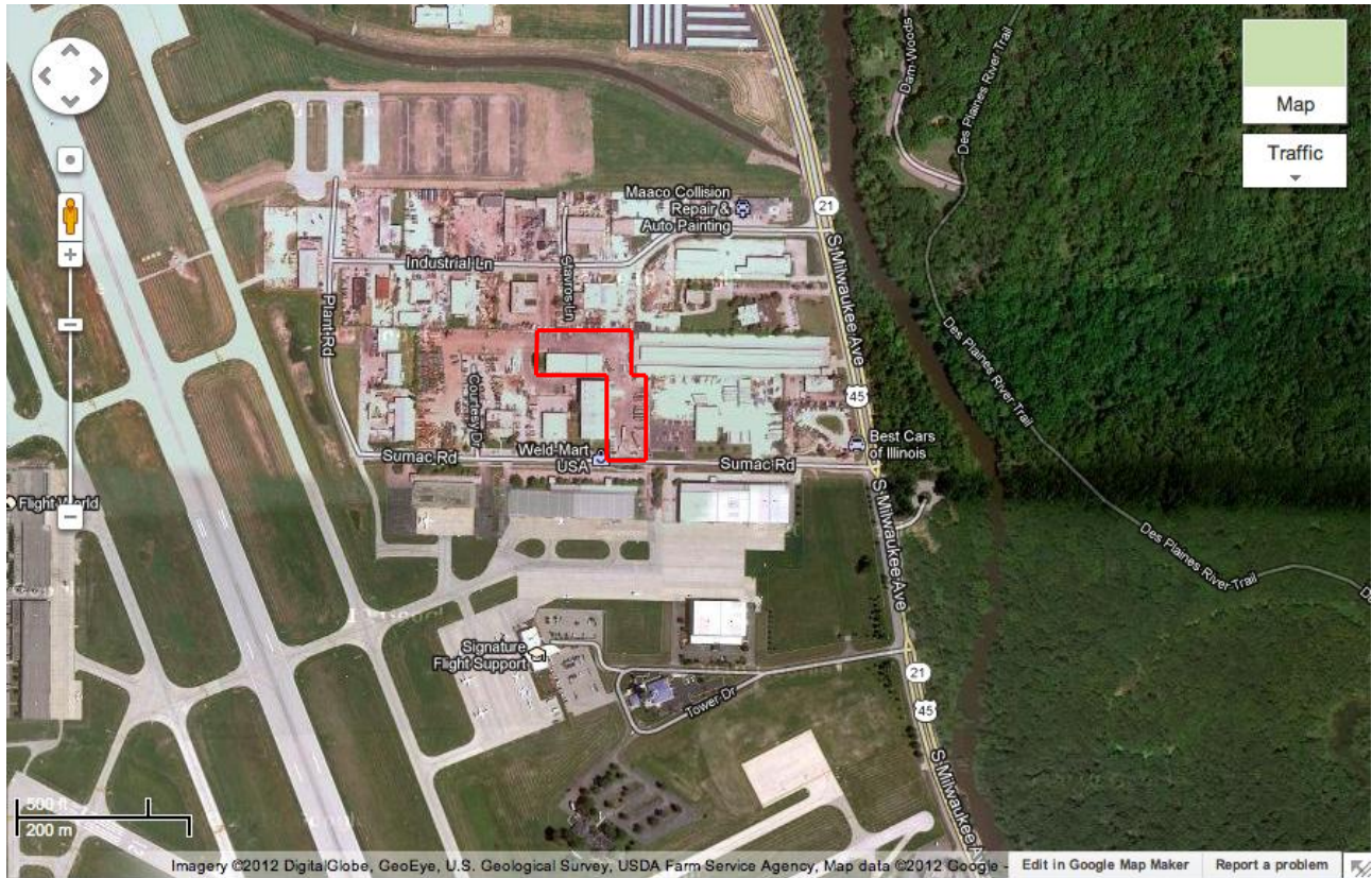
Google Maps image of the Waste Management-Northwest/Wheeling WTS (and adjacent industrial park buildings), operated by Waste Management.
